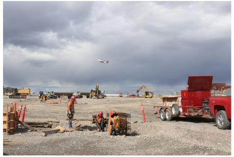
SCW North Apron Storm Drain Installation & Site Grading
