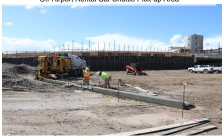
E Lot Curb & Gutter Concrete Placement
